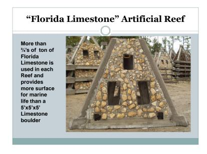
Walter Marine, "Reefmaker", developed and patented the process of attaching soft rock to a concrete structure. This produces a reef where the overall surface area of the rocks greatly exceed the surface area of the concrete structure, therefore attracting and providing habitat for all marine life associated with the natural reefs in the area, including
